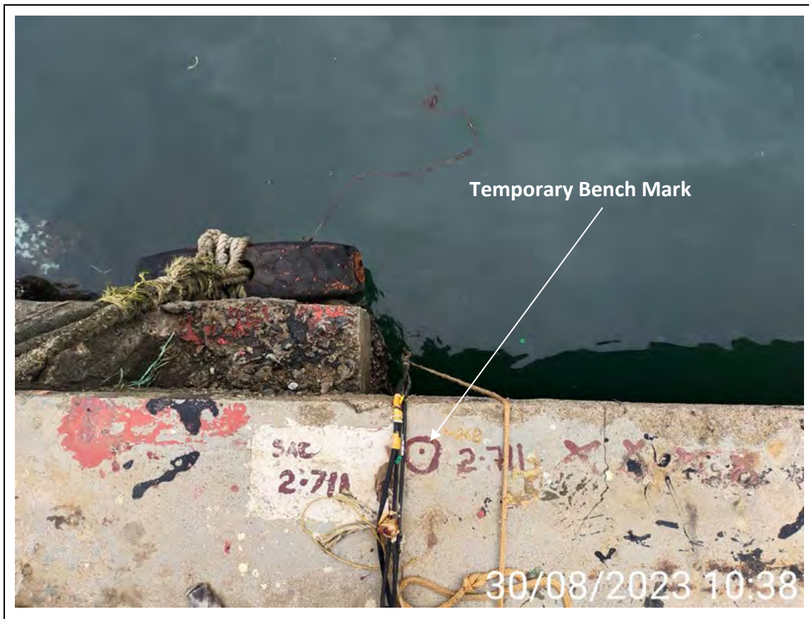
Figure 6-1: Location of TBM
