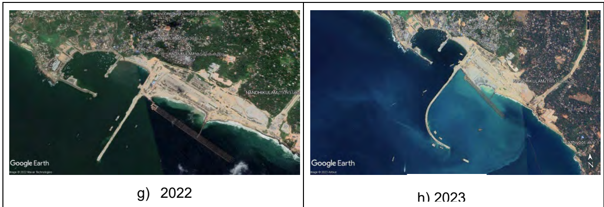
Figure 4-4 Different phases of breakwater construction.
