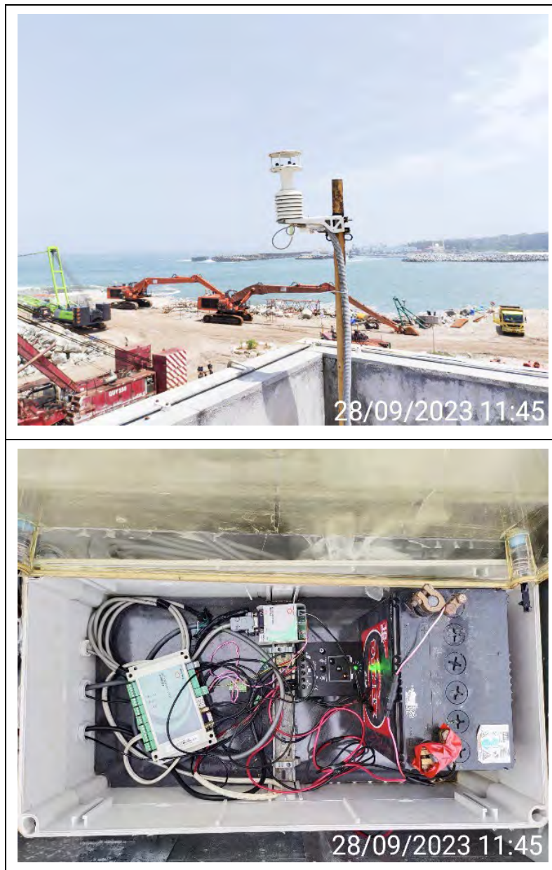
Figure 5-3: AWS on top of Port Control Office building
