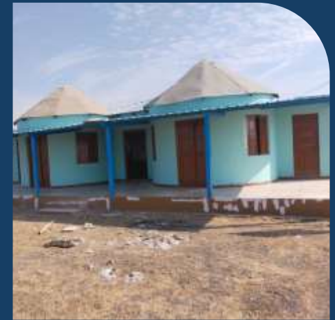
Renovation of Balwadi at Juna bandar & Luni bandar
