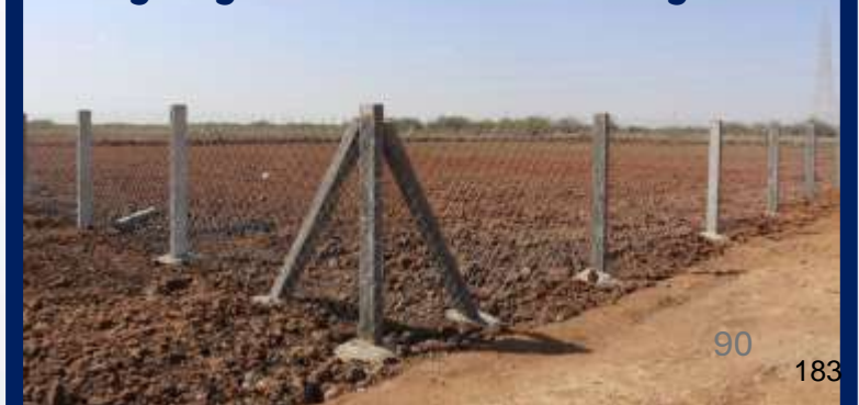
Ploughing of land & Wire fencing done!
