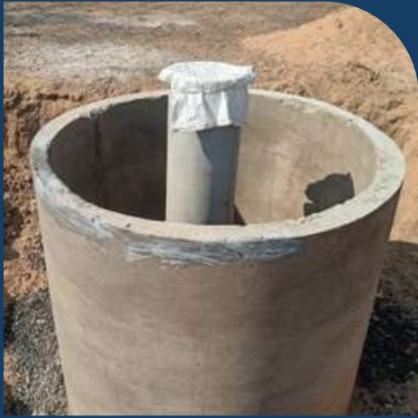
Construction of 21 Borewell Recharge in Nagmati River - 150+ farmer benefited
