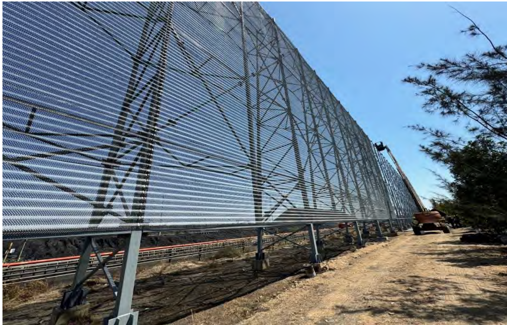
Ongoing Refurbishing work of Wind Screen
