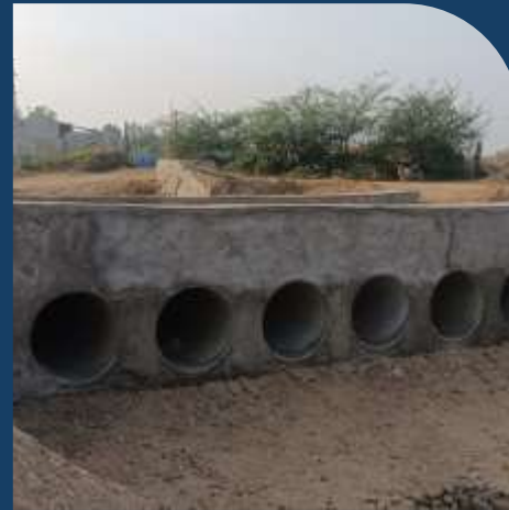
Construction of Pipe Culvert – 400+ Benefited
