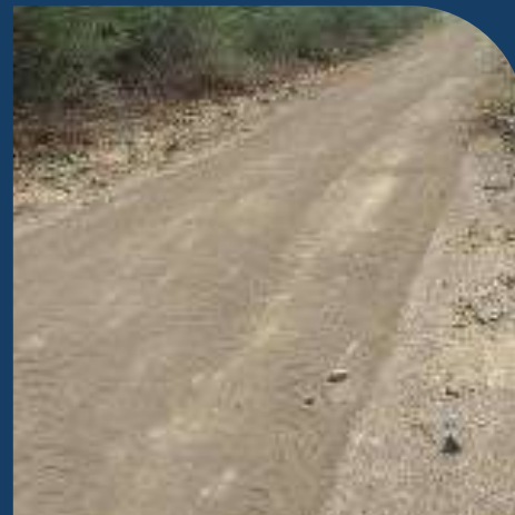
Renovation of approach road, Zarapara – benefiting 400 villagers
