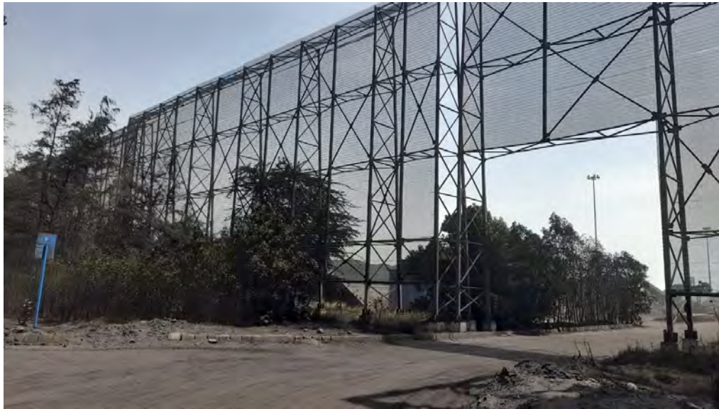
Installed Wind Screen
