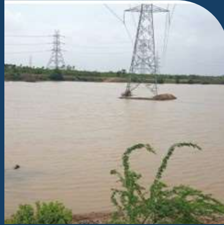
Check dam Desilting and restoration at Nana Bhadiya – 100+ farmers benefited
