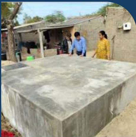
185 RRWHS construction is ongoing in various villages - will benefit 1300+ residents
