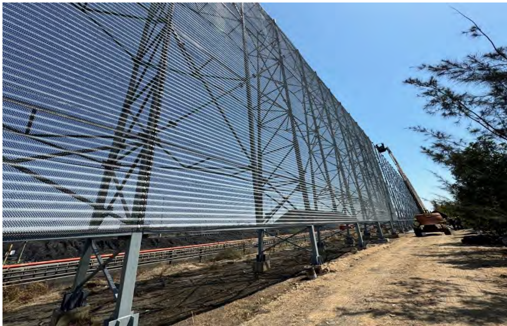
Ongoing Refurbishing work of Wind Screen
