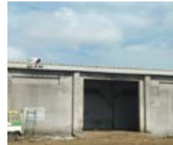
3 Villages - Renovation of Godown and Gauthala Shed
