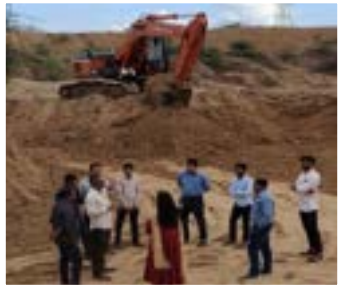
Restrengthening & Desilting of Check dam – 720+ Benefited
