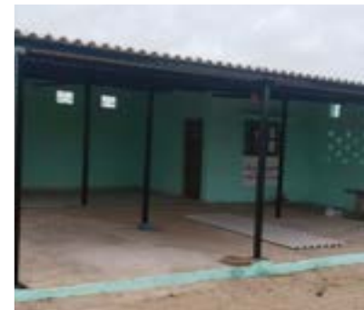
Renovation of Shed at Shekranpir Bhopavandh - 2000+ Benefited
