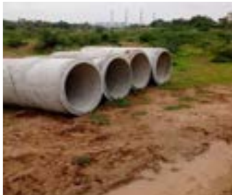
4 location Pipe Support – 4800+ Benefited
