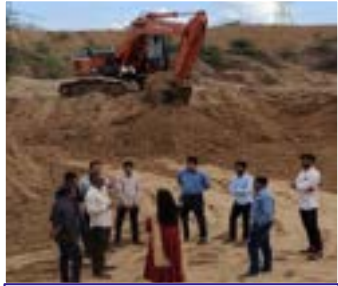
Restrengthening & Desilting of Check dam – 720+ Benefited
