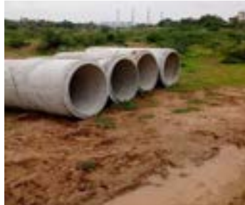
4 location Pipe Support – 4800+ Benefited
