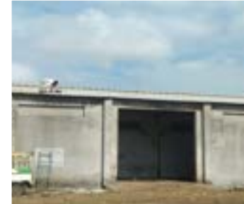
3 Villages - Renovation of Godown and Gauthala Shed
