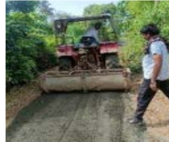
Renovation of Approach road Vadi Vistar at Mota bhadiya village.- 7200 Benefited
