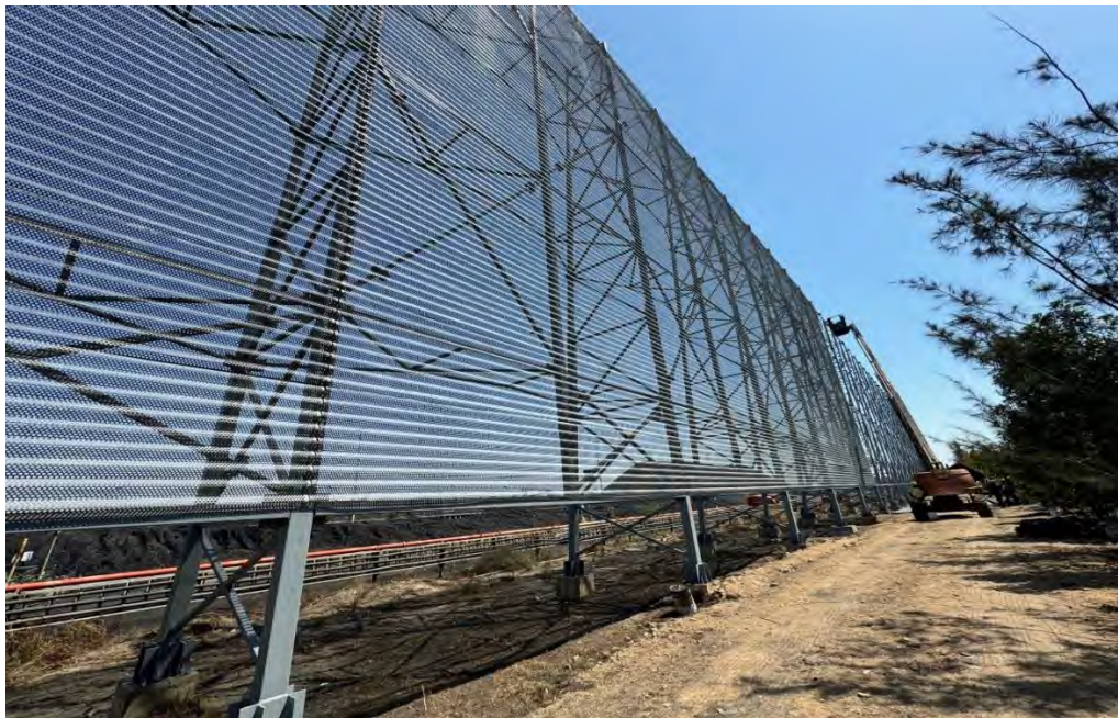
Ongoing Refurbishing work of Wind Screen
