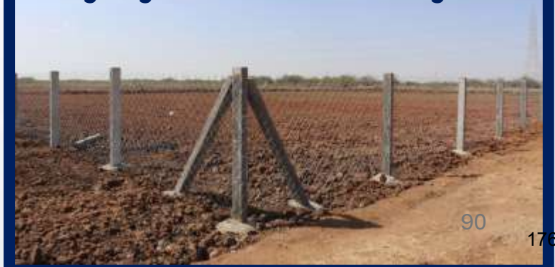
Ploughing of land & Wire fencing done!
