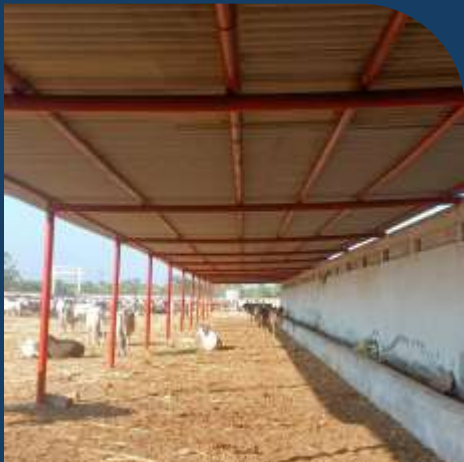
Gaushala Shed at Zarapara village – 400 cattle benefited
