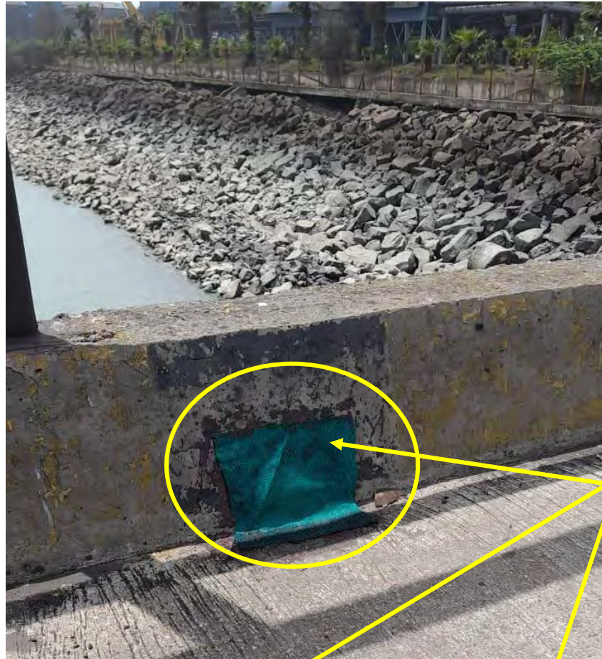
Filters at Jetty Outlet
