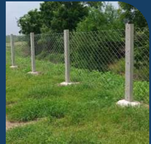
Construction of chain-link fencing at Mangra village – 300 people benefited
