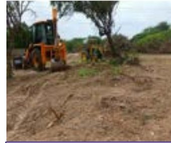
River Cleaning and JCB Support - 2250+ Benefited
