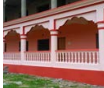
Renovation of High School at Zaarapa – 2200+ Benefited
