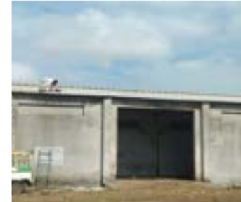
3 Villages - Renovation of Godown and Gauthala Shed
