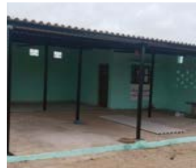
Renovation of Shed at Shekranpir Bhopavandh - 2000+ Benefited
