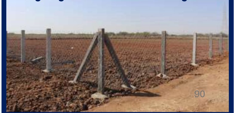
Ploughing of land & Wire fencing done!
