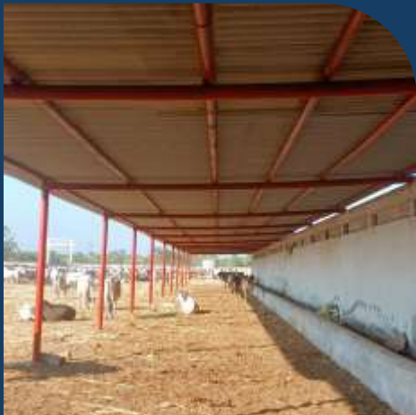
Gaushala Shed at Zarapara village – 400 cattle benefited
