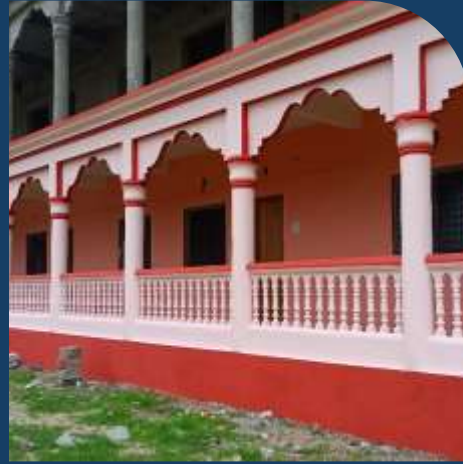
Renovation of High School at Zaarapa – 2200+ Benefited
