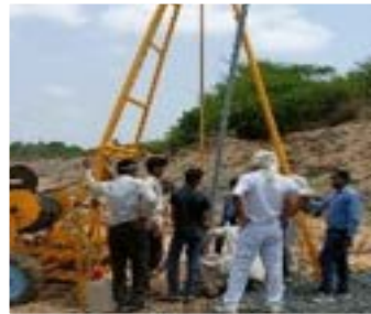
6 Percolation Bore well Recharge – 4000+ Benefited
