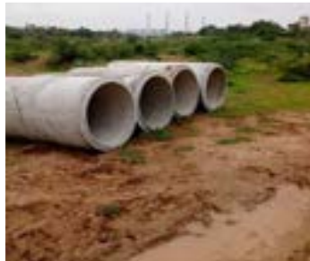
4 location Pipe Support – 4800+ Benefited
