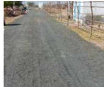
Road Renovation and Civil Maintenance Work at Fisherman Vasahat – 600+ Benefited
