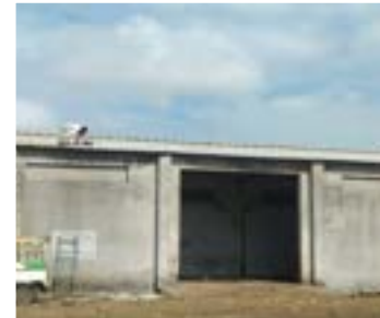
3 Villages - Renovation of Godown and Gauthala Shed
