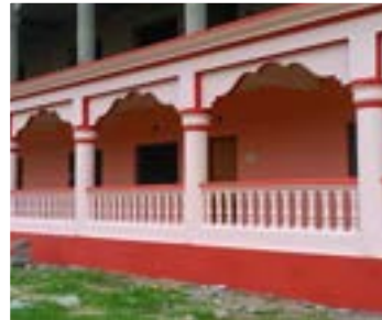
Renovation of High School at Zaarapa – 2200+ Benefited
