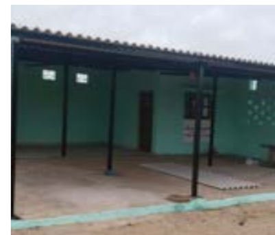
Renovation of Shed at Shekranpir Bhopavandh - 2000+ Benefited
