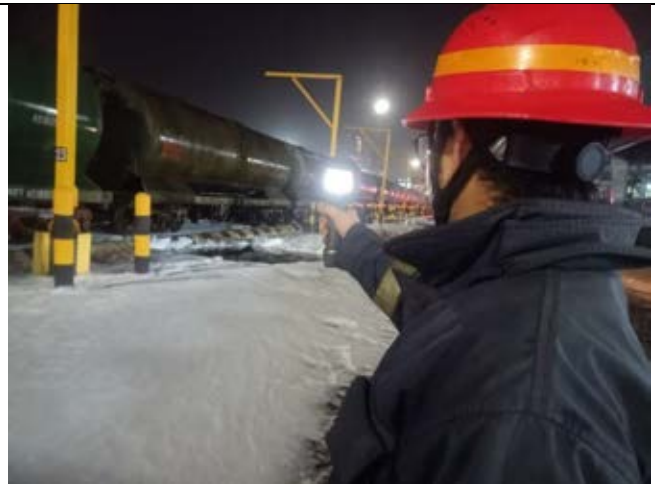
Wagon De-attachment & rail rack isolation work started by Railway services
