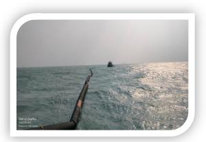
1015 hrs.: Completed lowering boom (5 section 250 m in length)
