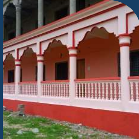
Renovation of High School at Zaarapa – 2200+ Benefited
