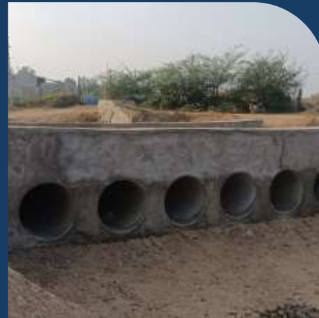
Construction of Pipe Culvert – 400+ Benefited
