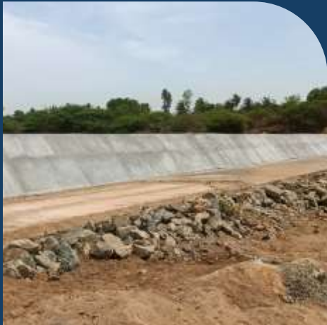
Renovation Check dam and CC road work at Nani Khakhar – 200+ benefited
