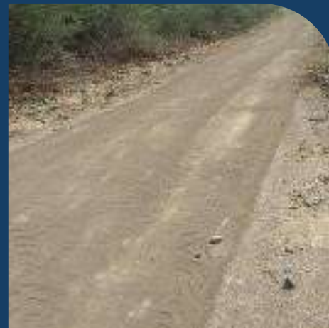
Renovation of approach road, Zarapara – benefiting 400 villagers
