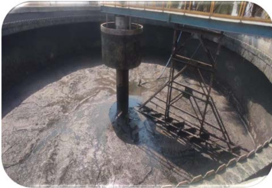
Secondary clarifier 1 and chlorination tank cleaning work
