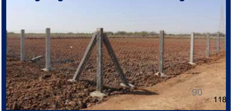
Ploughing of land & Wire fencing done!
