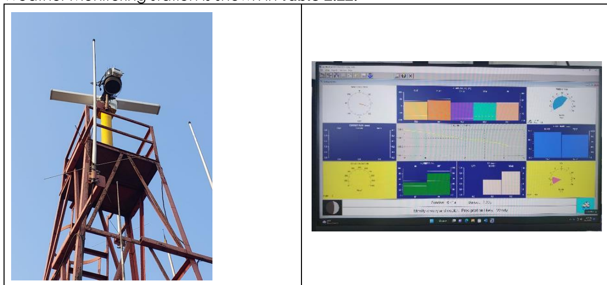
Figure 2:10 Continuous Weather Monitoring station at AKPL
