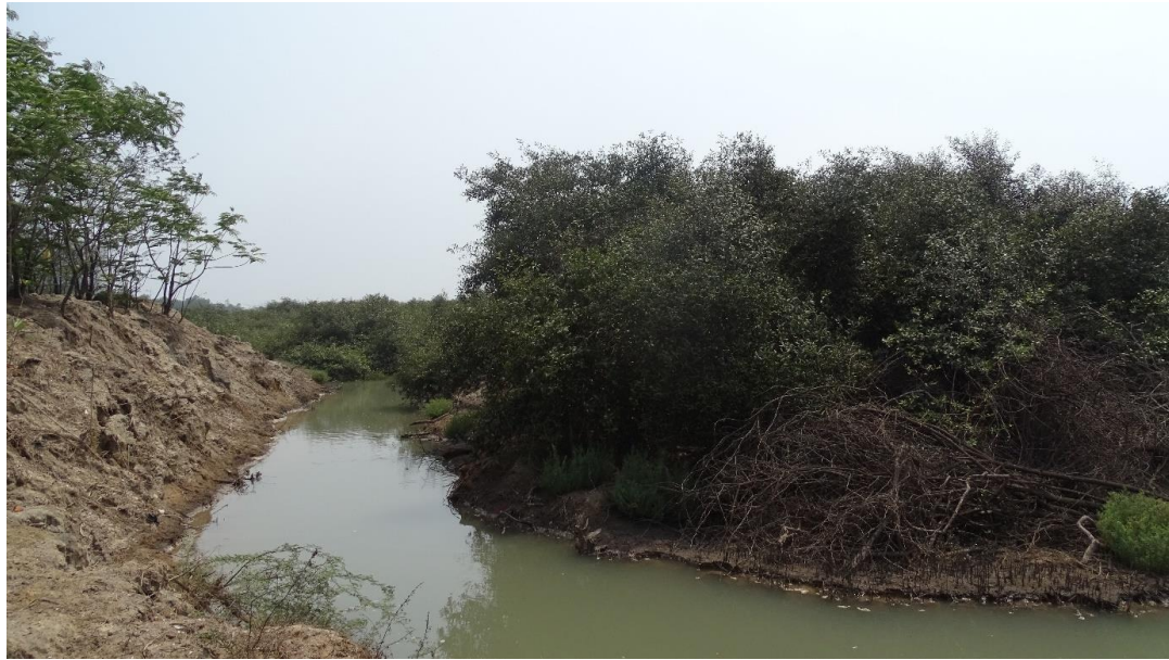
Proper drainage near Mangrove area of 50 Ha. developed by AKPL
