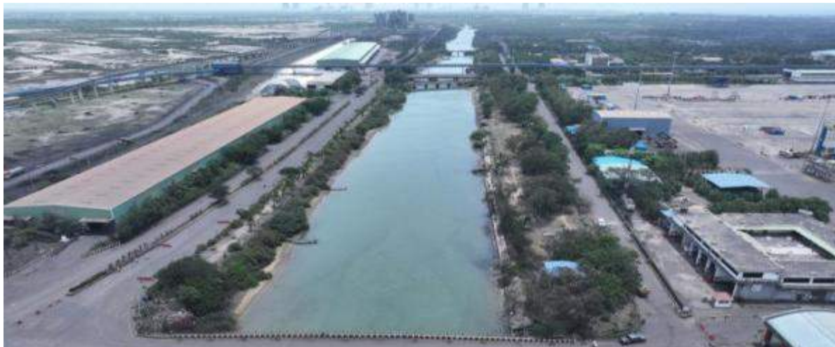
Greenbelt Protection to Buckingham Canal inside the port premises
