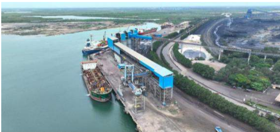
Closed hood conveyors & mechanical handling systems
