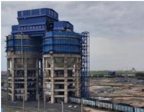
Silo for Railway rake loading
