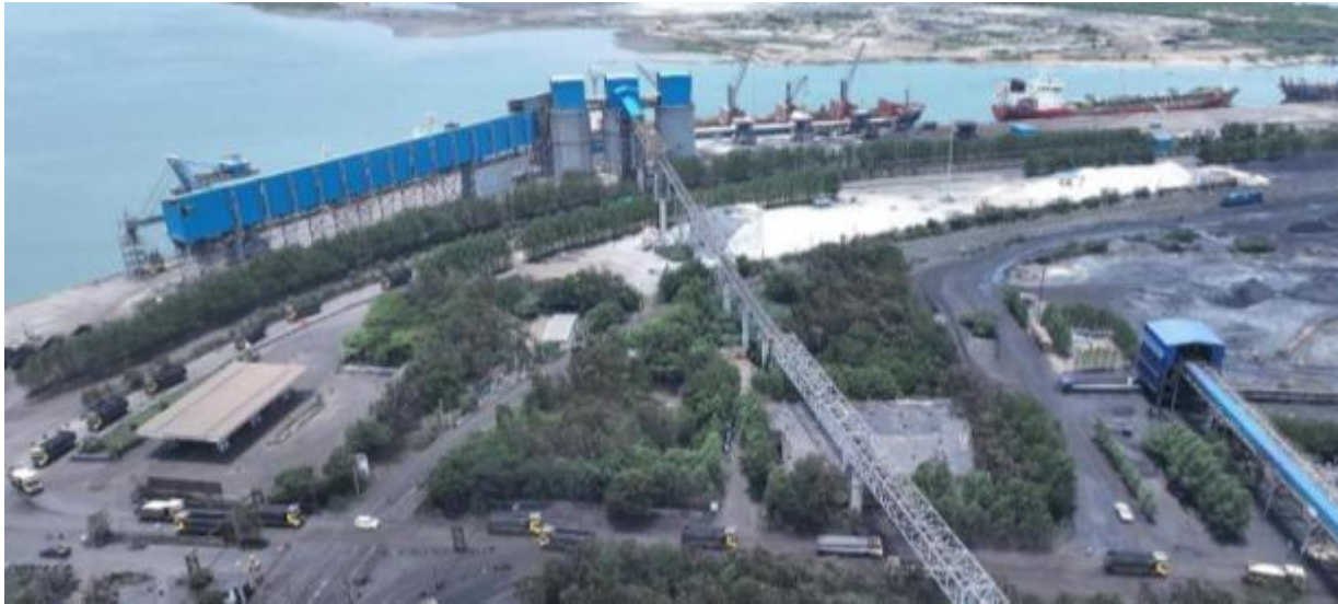
Conveyor Systems directly transferring cargo to industries
