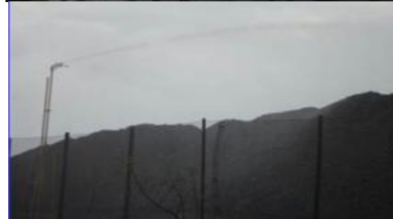
Mechanical Dust Suppression System – Water Sprinklers in Coal yards
