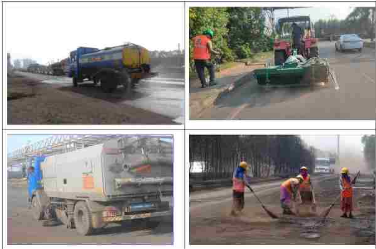
Figure 2:6 Vacuum Road Sweeping machines, Manual sweeping Sprinklers for Dry roads
