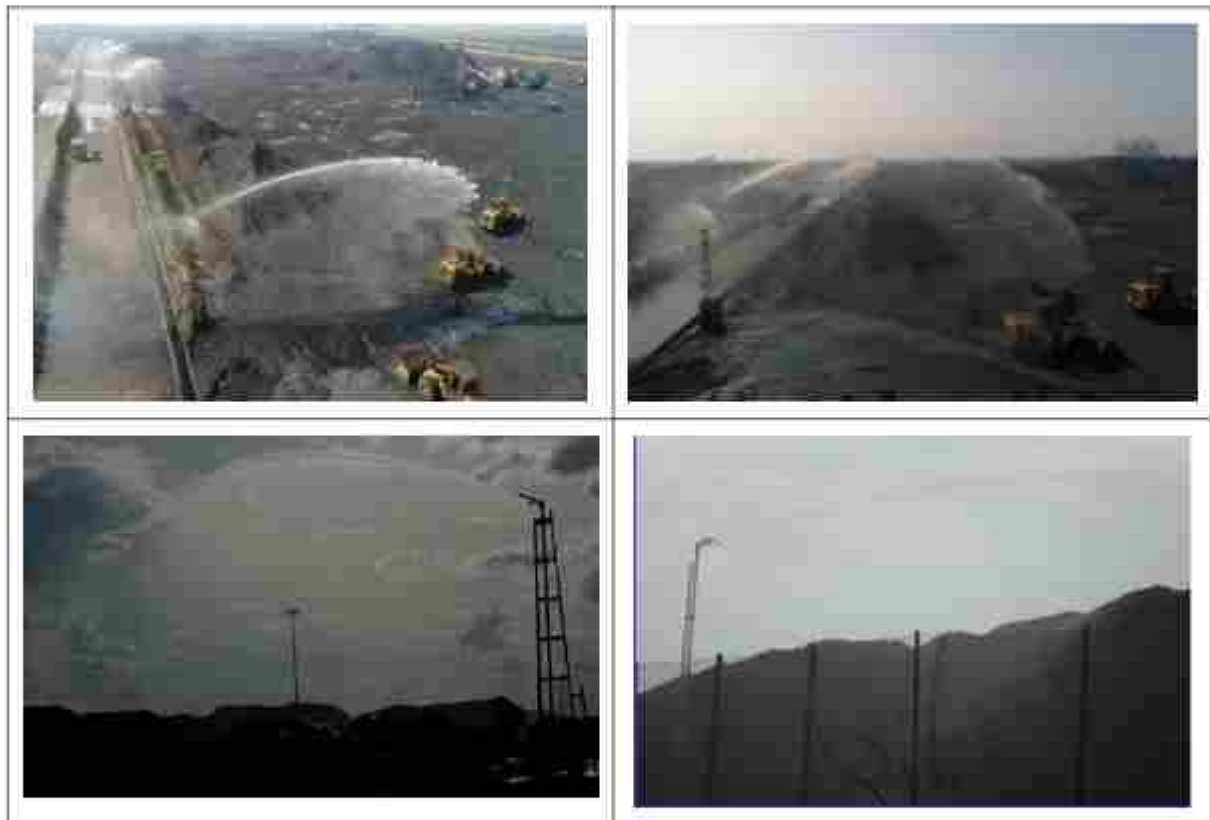
Figure 2:5 Mechanical Dust Suppression System – Water Sprinklers in Coal yards
