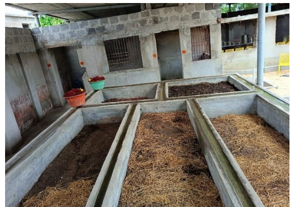
Vermi Composting Unit
