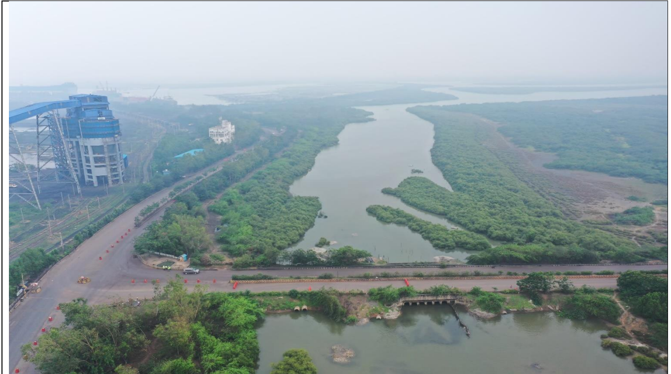
Greenbelt Protection to Buckingham Canal inside the port premises
