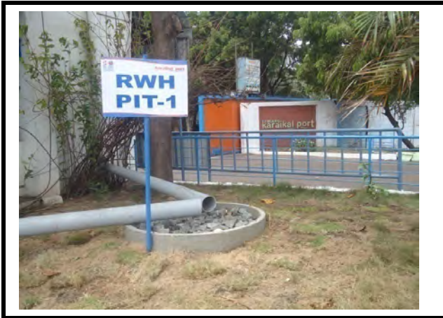
Rainwater harvesting Pits
