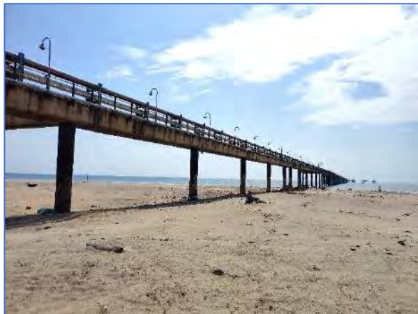
Deposition at north of north breakwater
