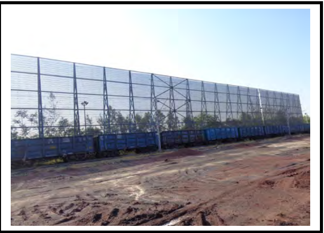
Wind Screen @ Coal Yards & Railway Sidings
