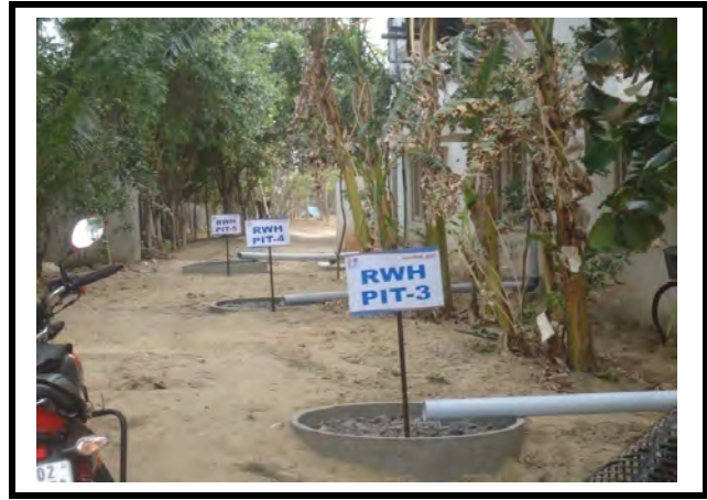
Rainwater harvesting Pits
