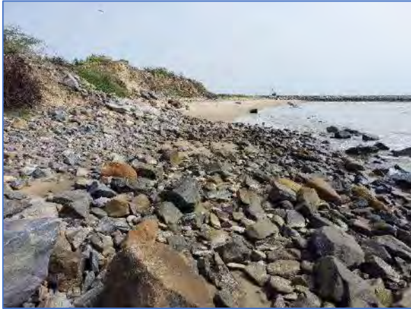
Erosion at south of south breakwater
