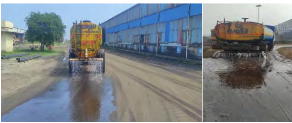
Road Wetting through Tankers / Tractors with spreaders
