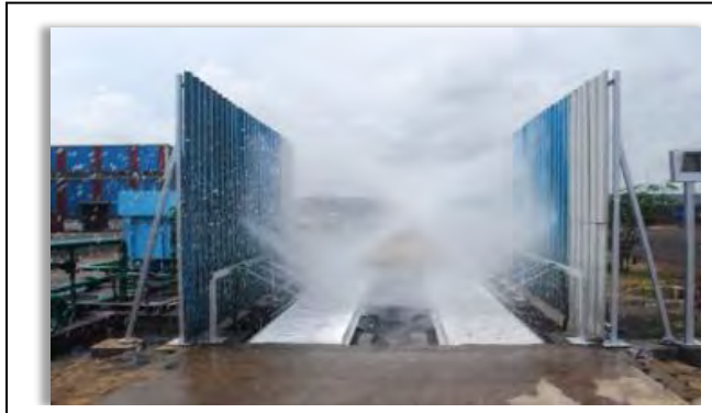
Annexure 3 -Automated Tyre Was System – Removes coal dust underneath of the vehicle
