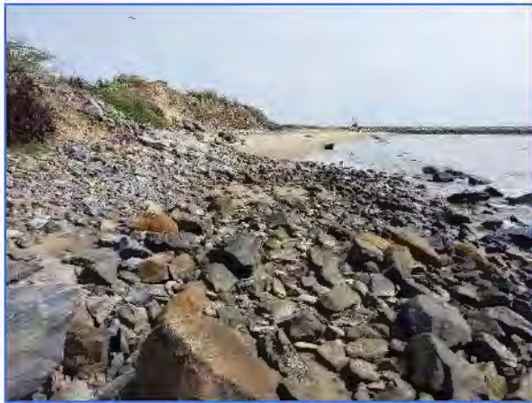
Erosion at south of south breakwater
