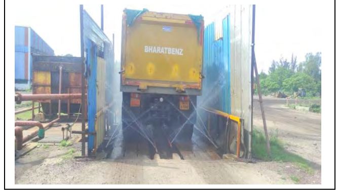
Annexure 3 -Automated Tyre Was System – Removes coal dust underneath of the vehicle
