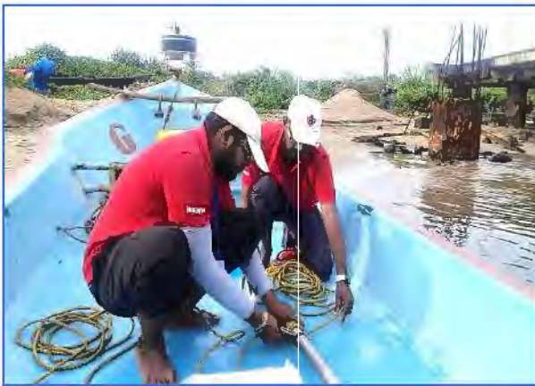
Installation of Transducer
