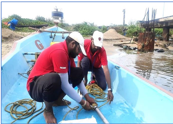
Installation of Transducer
