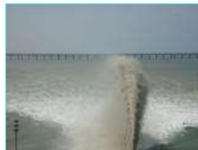
Placement of sediments for beach nourishment
