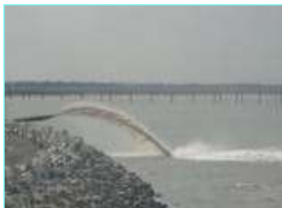
Placement of sediments for beach nourishment
