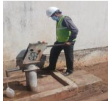
Bore well at Gangavaram (V)
