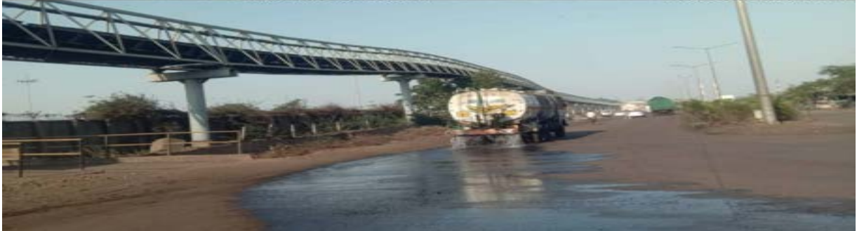
Water Sprinkling through Tanker
