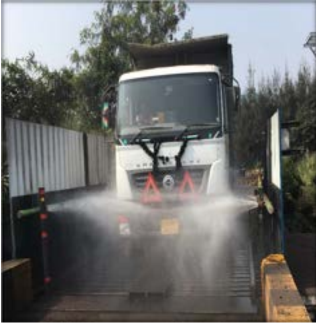
Truck Tyre Washing
