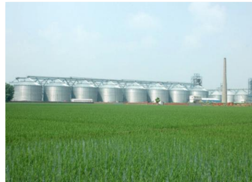
Moga (Punjab)- India's largest facility (2 lakh MT capacity)
